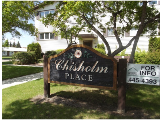
Chisholm Place: 10902 Winder Crescent
